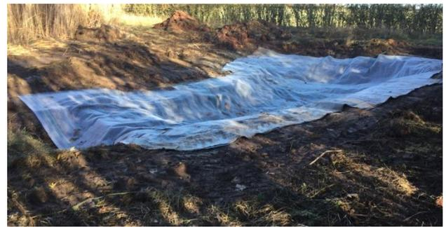
Dry pond, being lined after deepening and re-profiling
